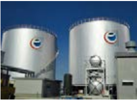
Sodegaura Asphalt Base
