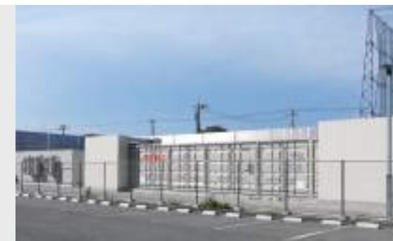
JAPEX Mihama Battery Energy Storage System
