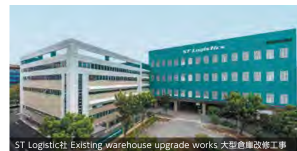
ST Logistic社 Existing warehouse upgrade works 大型倉庫改修工事
