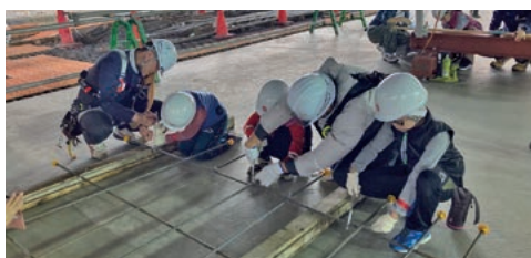
Hands-on work activity: Tying rebar together
