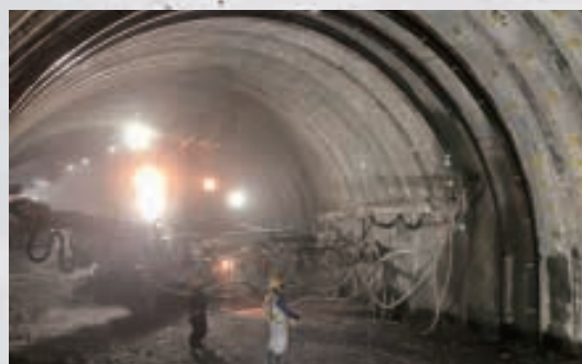
Spraying ultra-high-strength shotcrete
