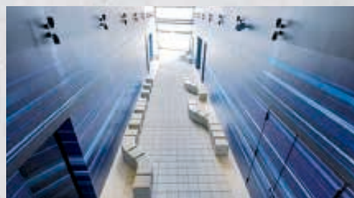
Carbon Pool concrete used for benches and flooring at the Future City pavilion at the Expo 2025 Osaka, Kansai, Japan.
