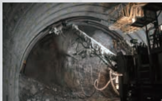
Installation of high-grade steel supports
