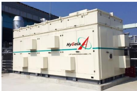
HyGeia-A : Small-Scale On-Site Hydrogen Generator
