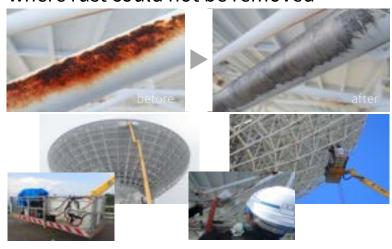
40m-tall parabolic antenna is constantly in motion, temporary scaffolding could not be set up, and the thick rust that is typical of coastal areas could not be removed.
