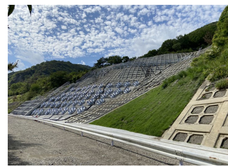
Slope reinforcement work in the Ako area of the Sanyo Expressway
