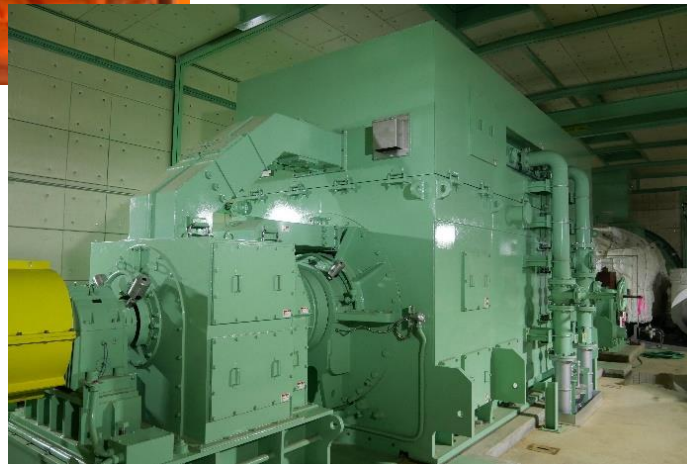
Left: PKS being fed into the fuel feed hopper Right: Steam turbine power generator
