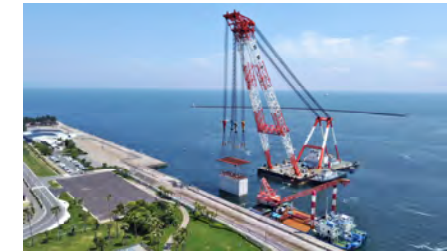
Quay wall construction
