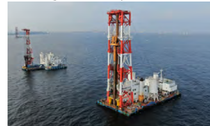
Offshore soil improvement work
