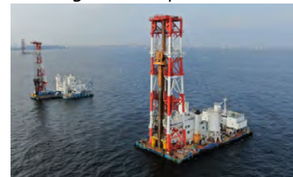
Offshore soil improvement work
