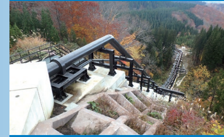
Wasabizawa Geothermal Power Plant production and return facilities construction
