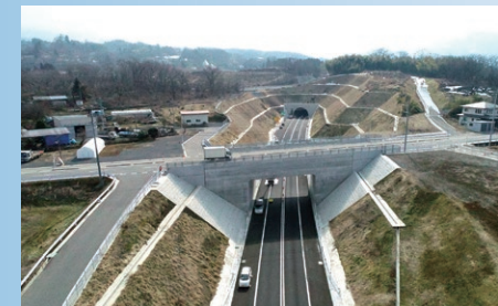
Tohoku-Chuo Expressway, Yamagatazao Tunnel construction
