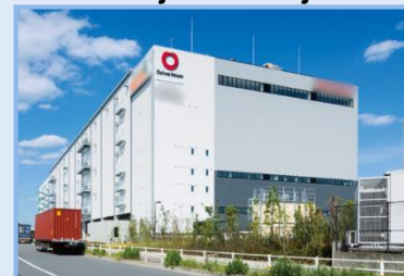
D Project Itabashi Shingashi
