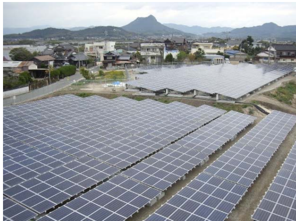
Ichigo Yamaguchi Aionishi ECO Power Plant (1.24MW)
