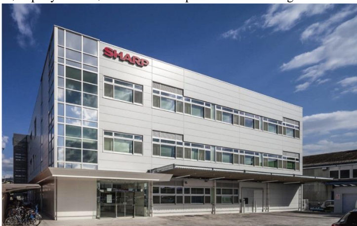
(Property number) OT-004 Sharp Hiroshima Building
