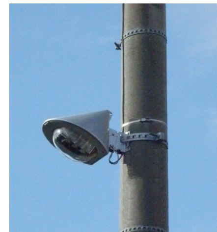
(施工例) LED防犯灯
