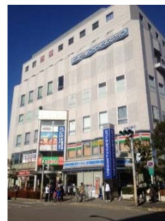
Inage Kaigan Ekimae Building
